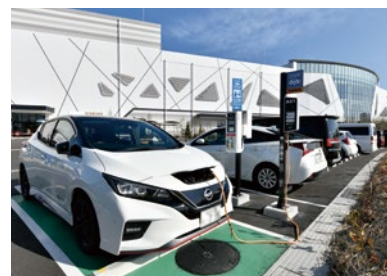
EV Charging Stations (AEON MALL Shinrifu South Wing (Miyagi Prefecture))
